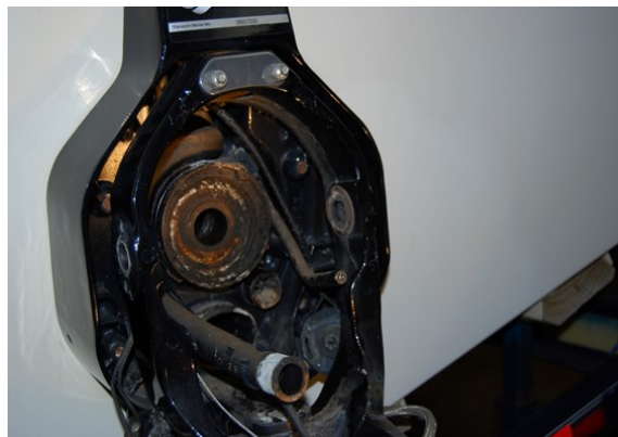
Drive shaft bellows neglect completely destroyed the gimbal bearing that used to be in the rusty housing.
